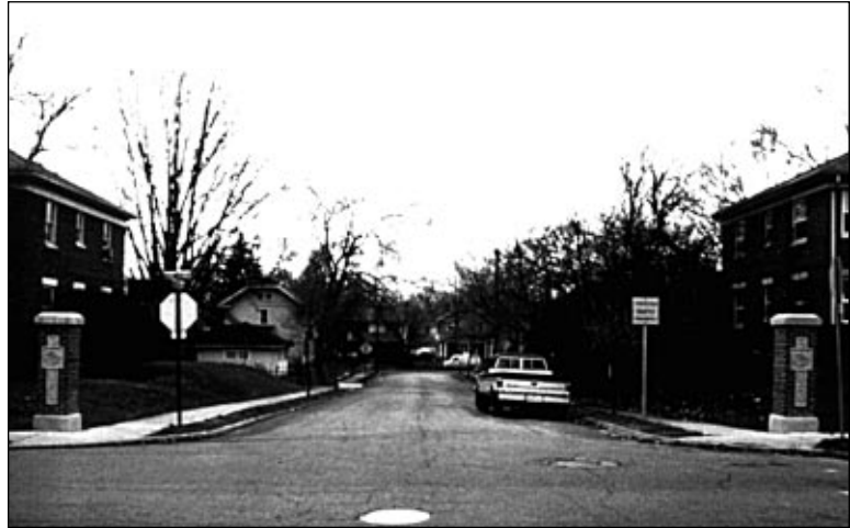
Figure II-16: Actual position of portals as installed.
