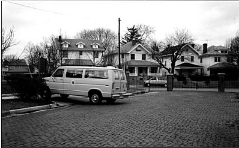
Figure II-14: Hammerhead turn at end of street.
