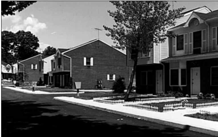
Figure IV-15: Residents' initial improvements to their front yards.
